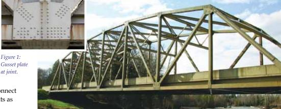
Figure 2. One of three WSDOT bridges used to develop the TEP for gusset plate evaluation.
