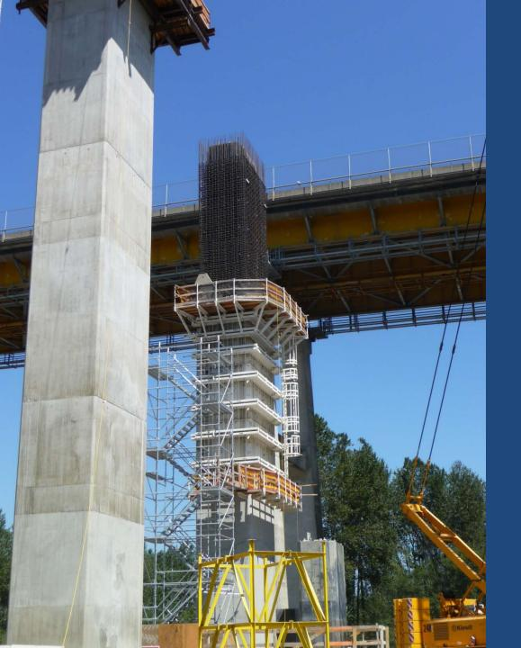
Formwork for column which is one of three for this pier.
