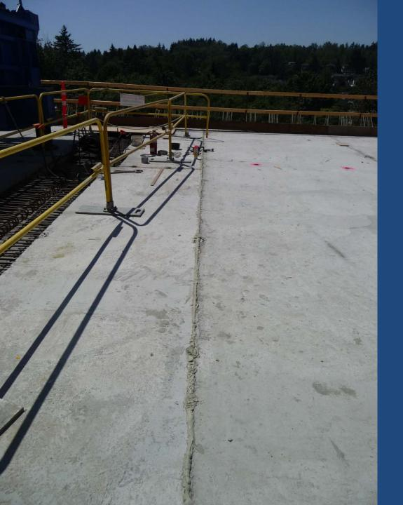
Joint between two precast segments
