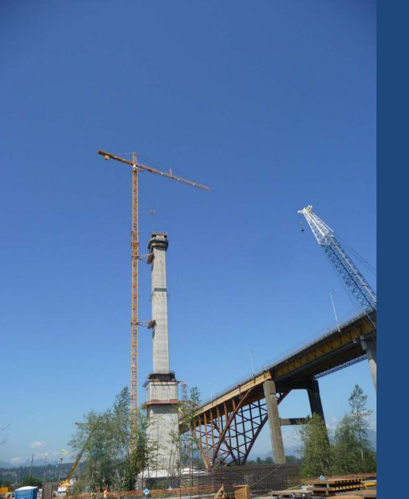
S1 pylon under construction—ultimate height 160 m (525 ft)
