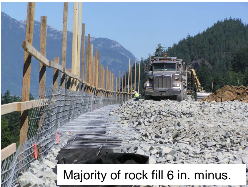
Face rock is 6 in. plus size (with a 2 ft width). Fabric separates the face rock from the remainder of the rock fill.
